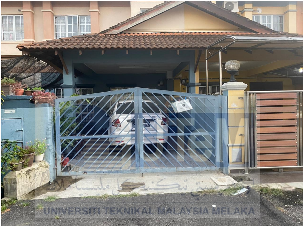
Figure 1.2 Example Of Current Situation In Home Property
