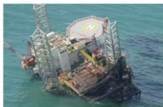
(c) Buckled/Collapsed oil rig platform
