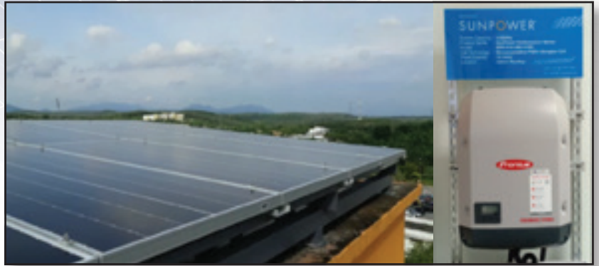
Figure 1: Installation (top view) and inverter model
