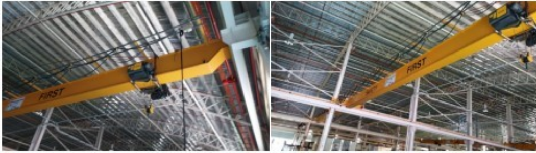
Figure 3.26 Cable and Crane that will be used for DIC
