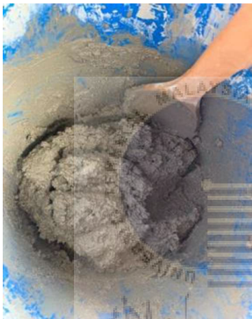
d) After adding water, the materials then proceed with wet mixing.
