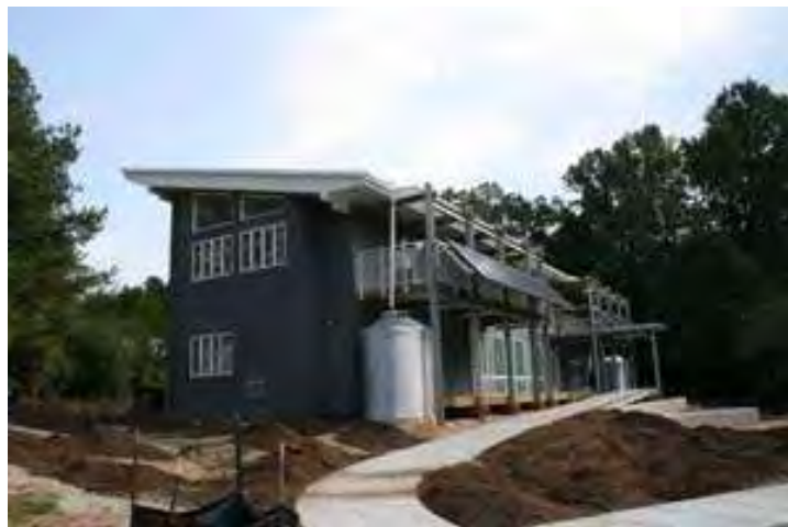
Figure 2.1(a): The Home Depot Smart Home
