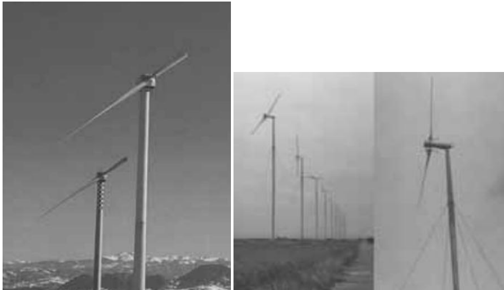
Figure 1-6: Single and twin bladed rotor design (Gardner, P)
