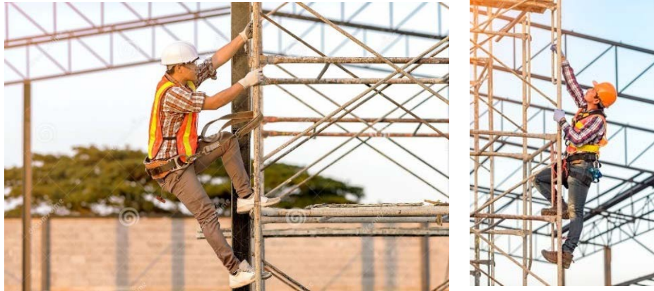
Figure 1.1: A worker climbing the scaffolds (Webb, 2017)
