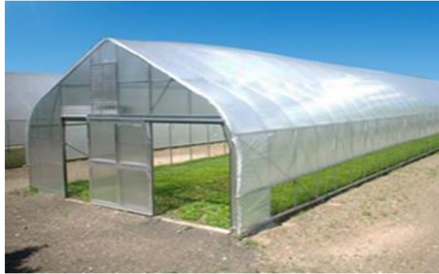
Figure 2.1 Galvanized Steel Pipe Frame Greenhouse
