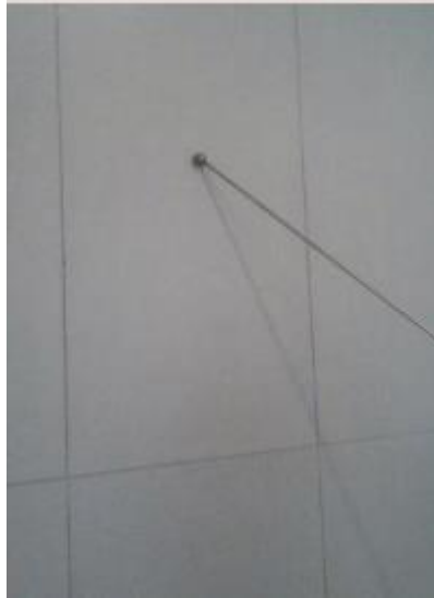
Figure 2.2: The metal rod used to detect the hollowness of floor
