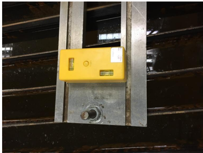
Figure 3.6: Leveling using water level
