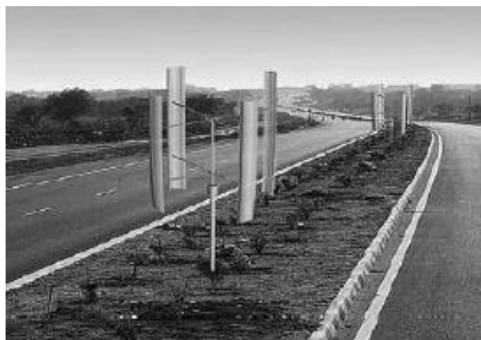
Figure 2.10: VAWT on middle of highway divider (Al-Aqel et al., 2016)
