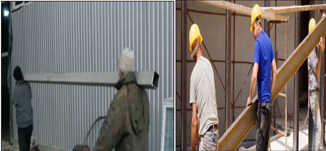
Figure 1.2: Manual handling long metal bar
