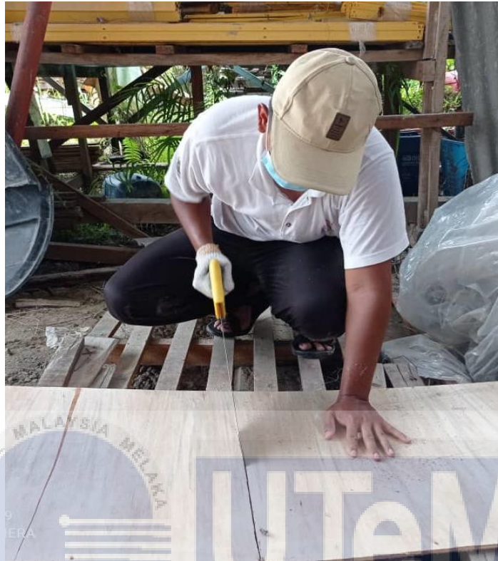
Figure 3.4: The cutting process for the plywood.
