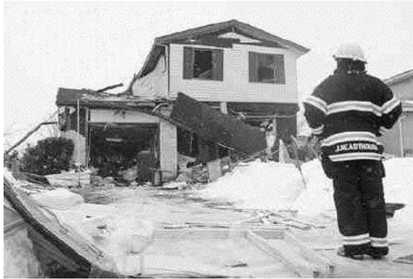
Figure 1.1: Damage that occurred due to LPG explosion
