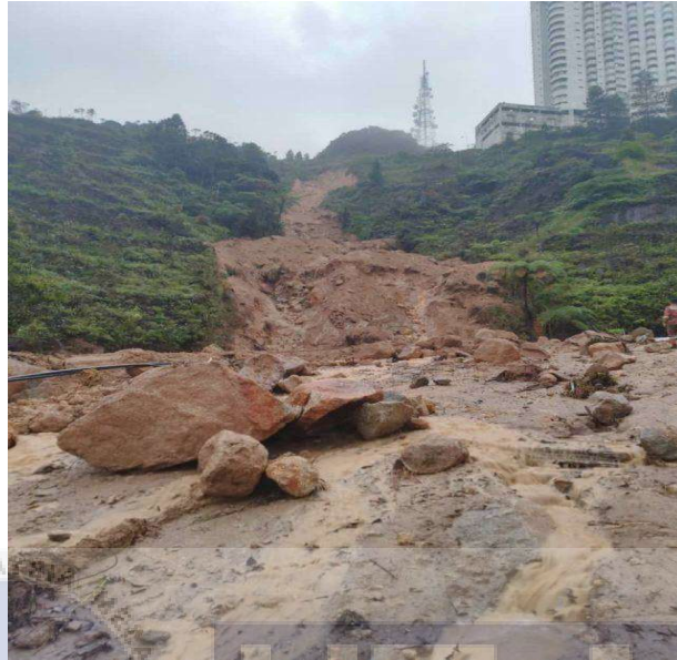
Figure 2.1: The major landslide in the Genting Highlands of Malaysia on 6 November 2019.
