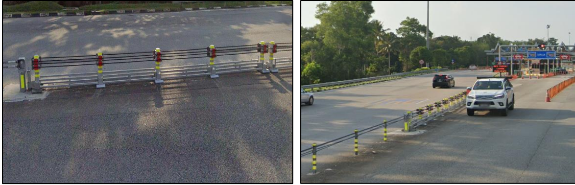
Figure 1.1: Current moveable fence at exit toll Ayer Keroh, Melaka
