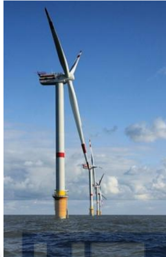
Figure 2.2: Example of Horizontal Axis Wind Turbine.
