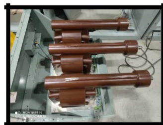
Figure 2.4: Voltage Transformer (VT)
