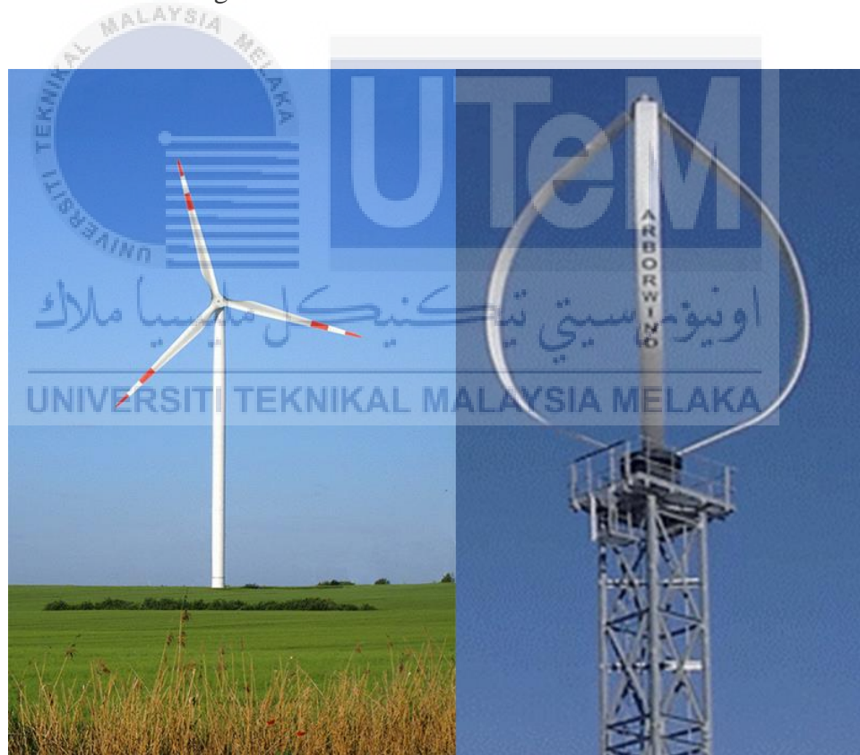
Figure 2.6.1: Horizontal Axis Wind Turbine (Left) and Vertical Axis Wind Turbine (Right) [2]
