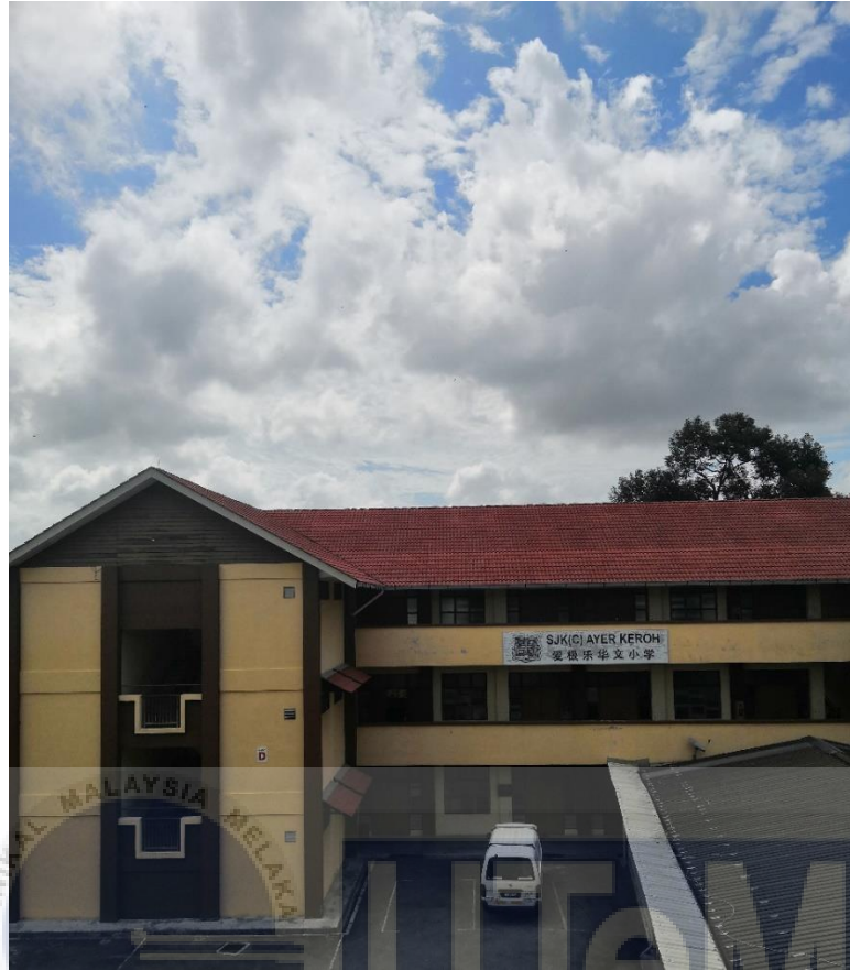
Figure 4.3: Target building for the RWH system.
