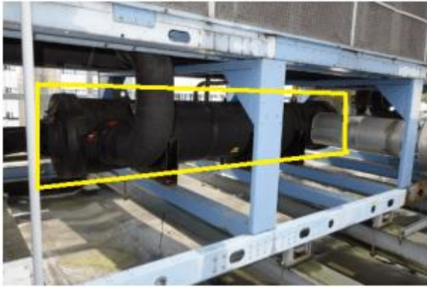
Figure 2.2(a) : Evaporator on an air cooled chiller
