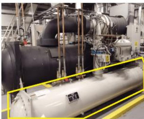
Figure 2.4(a) : Water cooled chiller condenser
