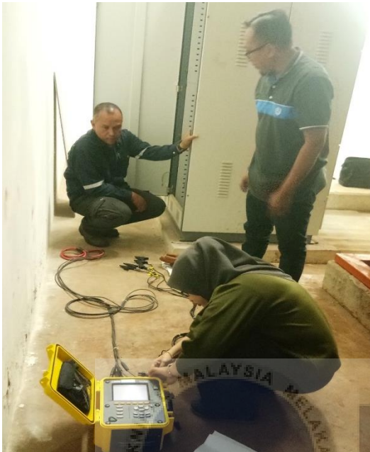
Preparing the data power logger to connect into power control unit.
