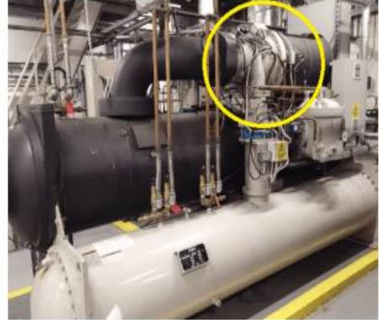
Figure 2.3(b) : Centrifugal type compressor
