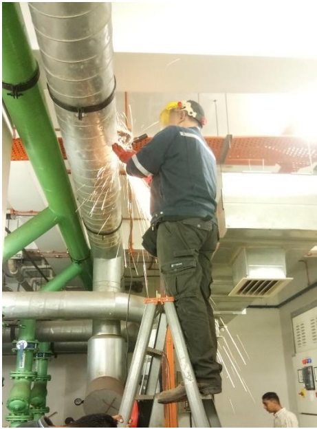
Welding to remove the insulated flowrate pipe for attach the ultrasonic power meter.
