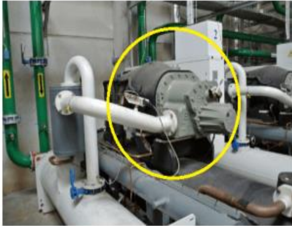
Figure 2.3(a) : Screw type compressor
