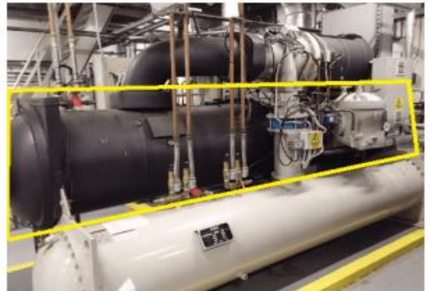
Figure 2.2(b) : Evaporator on a water cooled chiller
