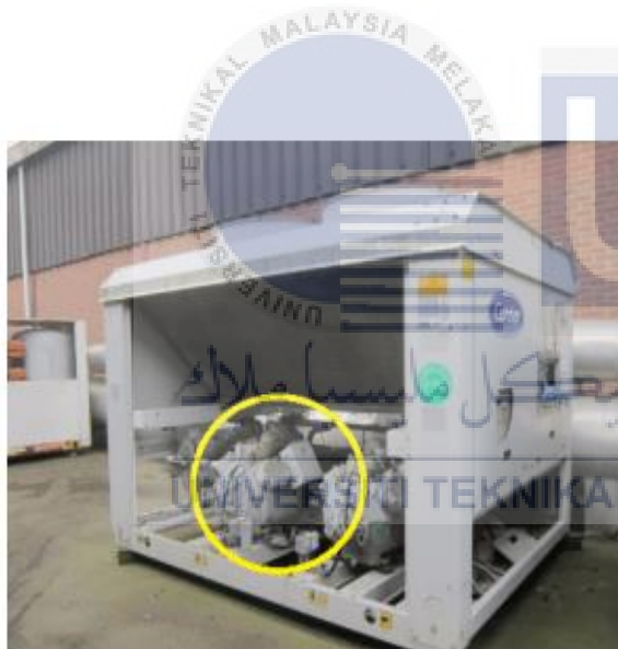
Figure 2.3(c) : Reciprocating type compressor
