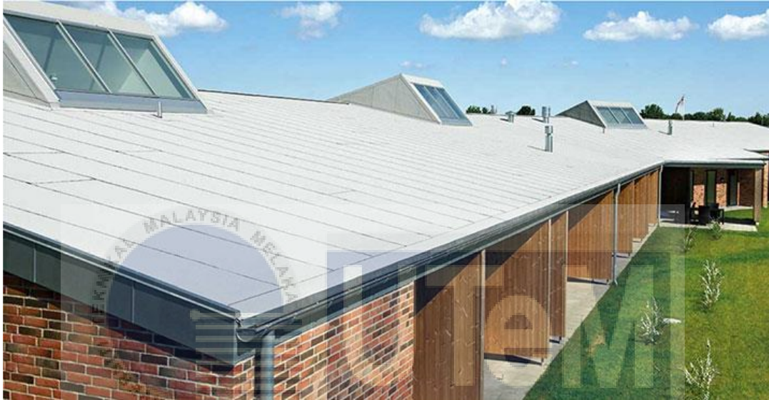
Figure 4.60: Cool roof system by BMI Group
