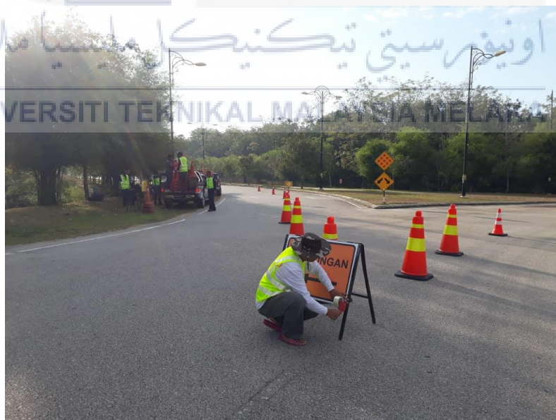
Figure 3.35: The situation after the cones and signboards have been set up
