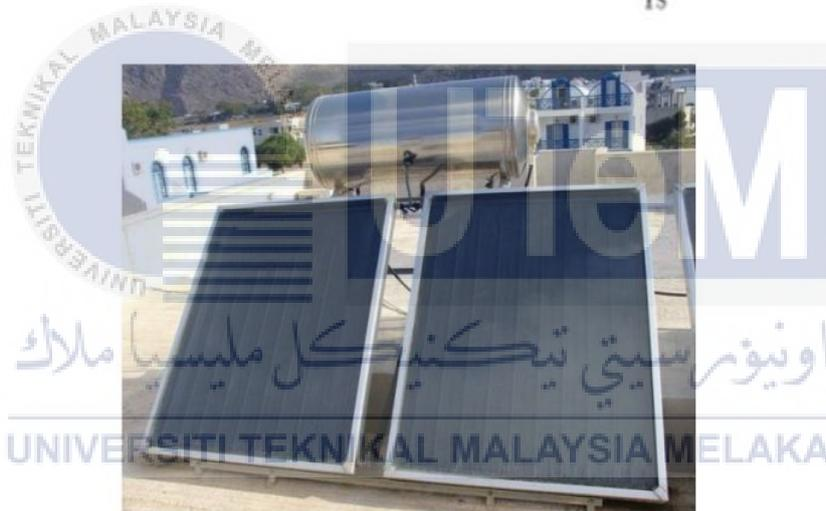
Figure 3.3.3.1(a) Actual model of Flat Plate Collector in Karaikudi.
