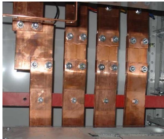
Figure 2.3.2: Type of busbar
