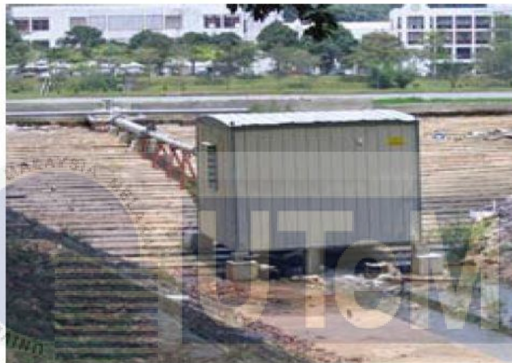
Figure 2.5: Pico hydro power plant at UKM, Bangi.
