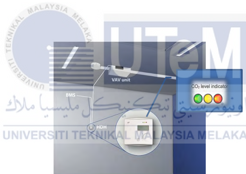
Figure 4.34: HDH transmitters operating diagram (Retrieved from http://www.produal.com/news/new-co2-transmitter-hdh-pir-pir-functionality-room-occupancy-detection/ )
