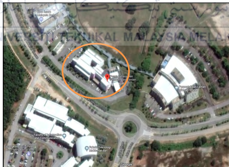
Figure 3.1: PBPI building from Satellite view [Source: Google Maps]
