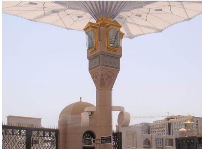
Figure 2.2: The world's largest evaporative cooling system in Medina, Saudi Arabia (Leo Rasmussen, 2013)
