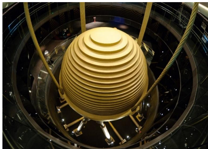
Figure 2.5: Taipei 101 tuned mass damper [Source: (Du Plessis, 2012)].
