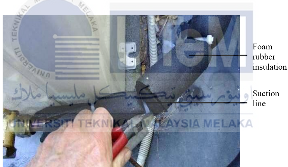
Figure 5.2.1: The insulation of thermocouple to the suction line
