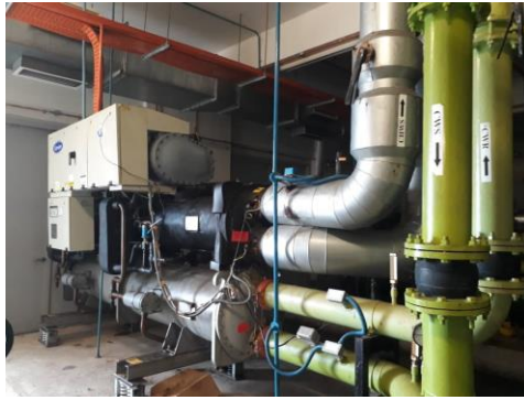
Figure 4-7: Chiller System
