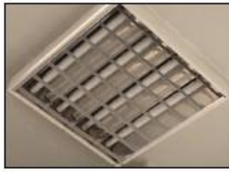
Figure 4-18 4 × 18W T8 Fluorescent DAVIS Light
