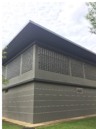
Figure 4-6: Chiller of FKE Space
