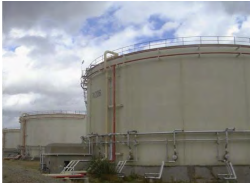
Figure 1.1 Steel Tanks in Practical Engineering (Zhao and Lin, 2014)
