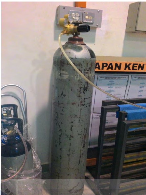
Figure 3.14: Nitrogen Gas Tank
