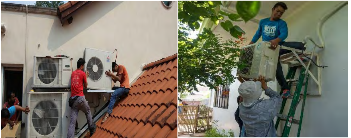
Figure 1.1: Manpower to lifting outdoor unit
