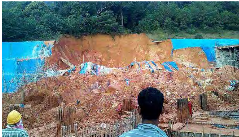
Figure 1.2: Landslide occur in Tanjung Bungah
