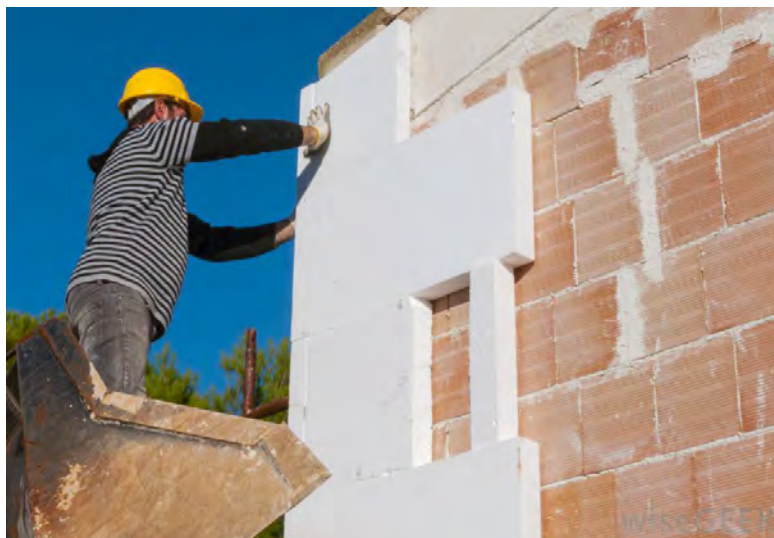
Figure 1.1: Extruded polystyrene foam as building wall insulation (KIMMU, 2017).
