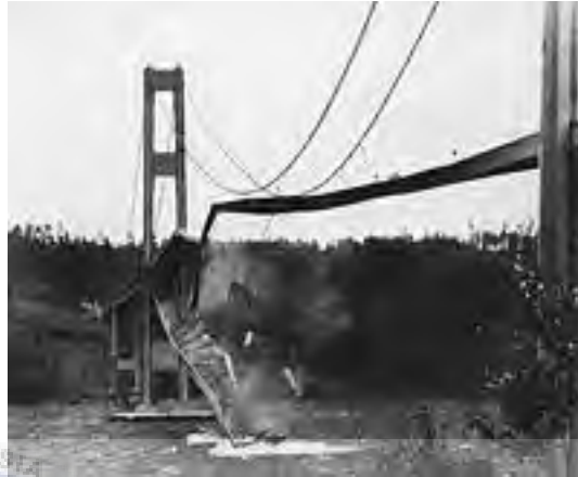
Figure 1.1: Collapse of Tacoma Bridge (Ellison, 2015).
