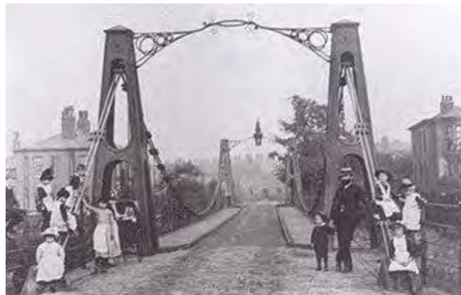
Figure 1.2: Broughton Suspended Bridge after Rebuilt (Dan, 2016).
