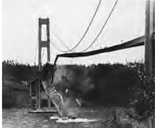
Figure 1.1: Collapse of Tacoma Bridge (Ellison, 2015).
