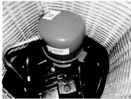
Figure 2.3 : Compressor mounted in housing
