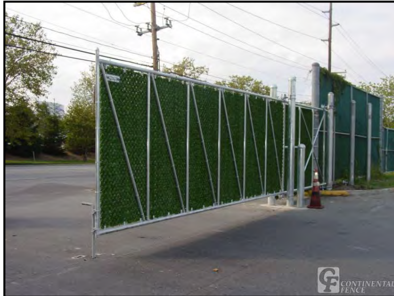
Figure 2.2: Cantilever slide type fence (Source: Security/Fences/Gates,n.d.)
