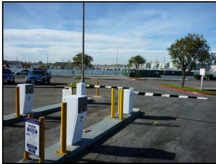
Figure 2.5: Barrier arm fence (Source: Parking/Barrier Gates,n.d.)
