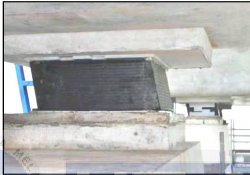
Figure 2.6: Rubber bearing under Penang Second Bridge (M. Salim et al., 2016)
