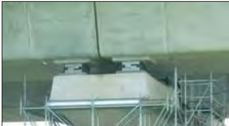
Figure 2.4: Application of LR-MS on Penang second bridge.
