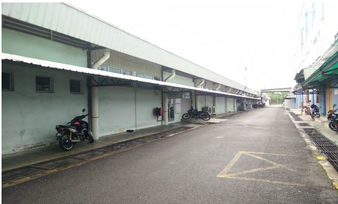
Figure 1.0: The View of Factory 2, Faculty of Engineering Technology, UTeM
