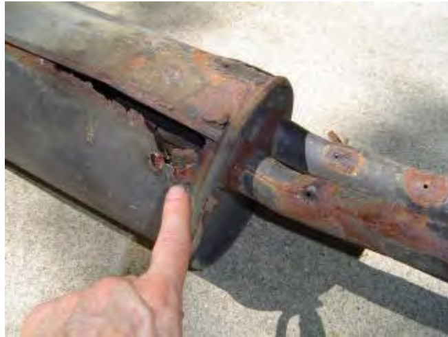
Figure 1.2: Corrosion on muffler leak
