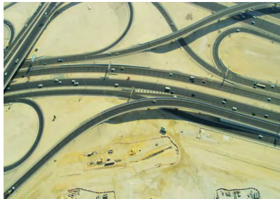
Figure 1. 4: Road construction of Dubai in Arab [9].
