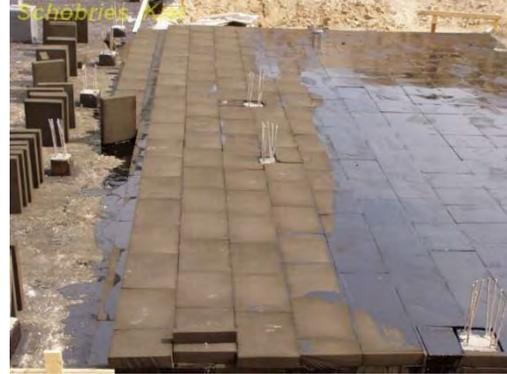
Figure 1.2: Foam Glass use at floor
