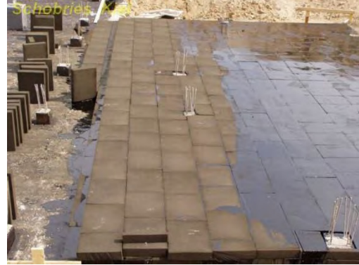
Figure 1.2: Foam Glass use at floor
