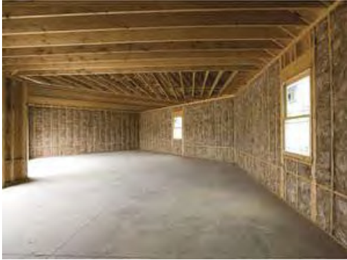
Figure 1.1: Glass wool use at wall
