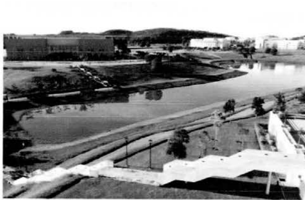
Figure 1.2: Area of the lake bank
