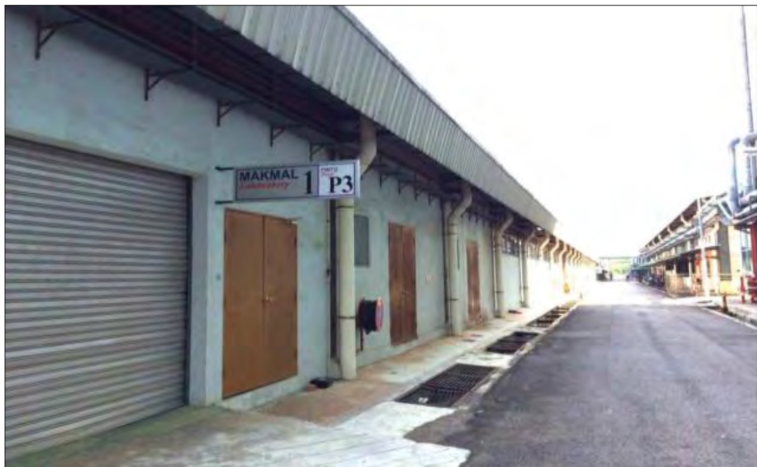
Figure 1.1: The view of Factory 1, Faculty of Engineering Technology, UTeM
